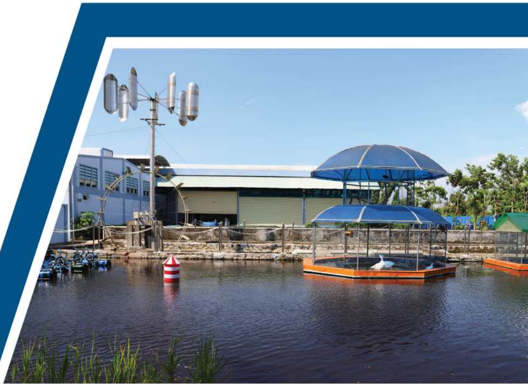
Lake area for regulating wastewater treatment
